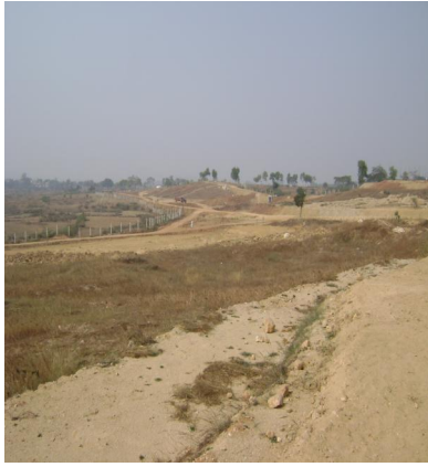
Initial Photograph of the site before Execution of MGNREGA Work
